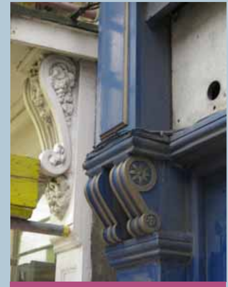
Historic details often survive beneath later alterations to shop facades.
