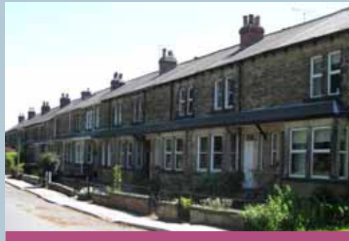
Sandringham Road. The window bays have been linked with a pentice along the length of the row.
