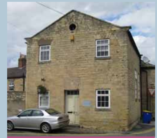
The former Non-Conformist chapel on Victoria Street, built in 1817.
