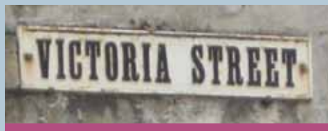
Cast iron street name plate in need of some maintenance.
