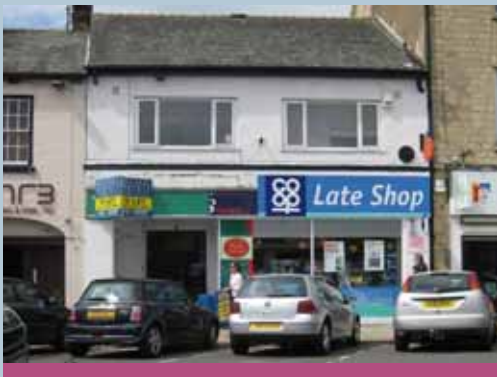
Over-dominant fascias detract from the character of the streetscene.
