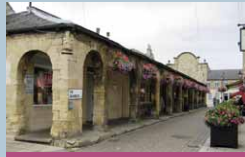
The Shambles creates a distinctive shopping environment, potentially attractive to tourists and regular shoppers.
