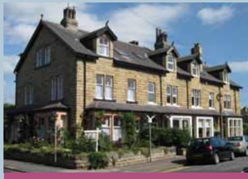
A more vertical emphasis is found on Caxton Street, with prominent chimneys, gable finials and dormers.
