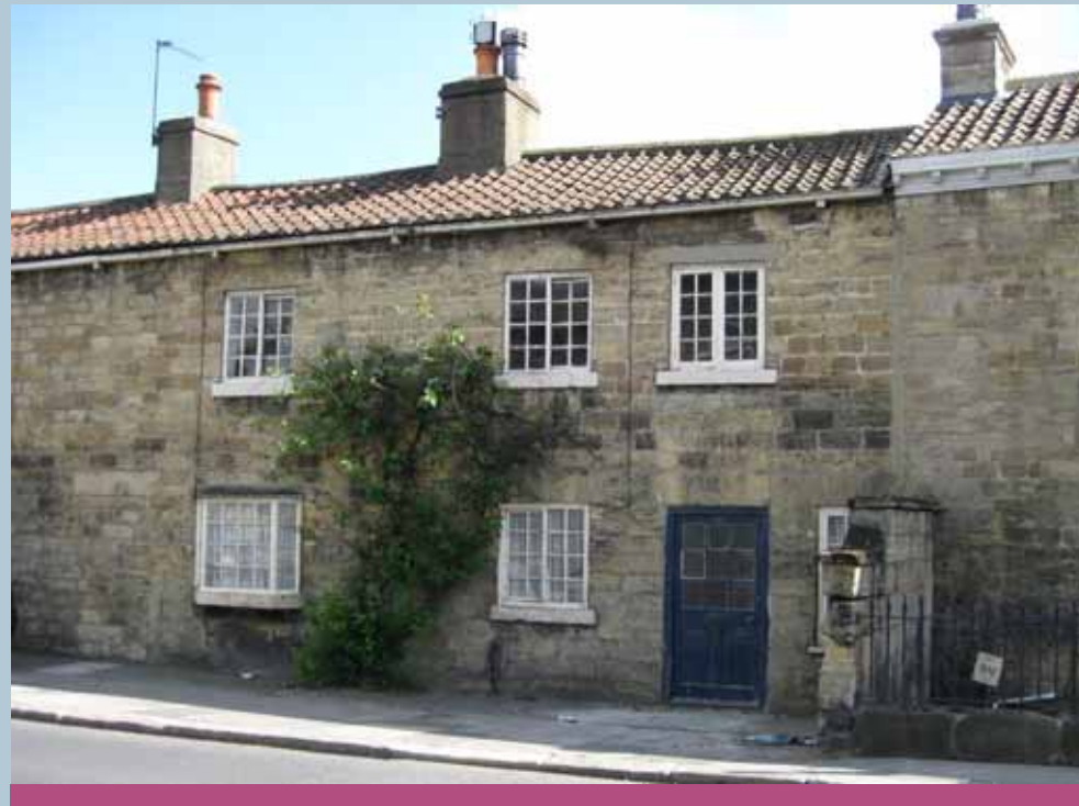
Vernacular houses constructed of local oolitic magnesian limestone with pantile roof and horizontally-sliding sash windows.
