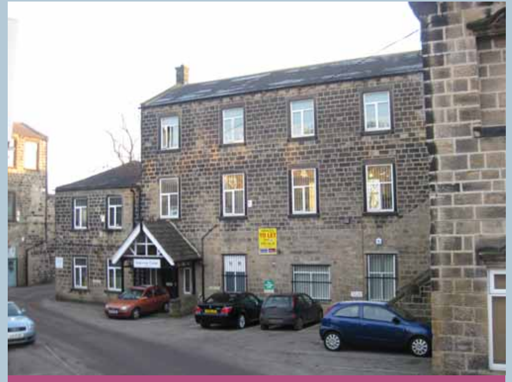
Three storey construction, regularly coursed sandstone, and regular fenestration patterns all contribute to the historic character and appearance of the conservation area
