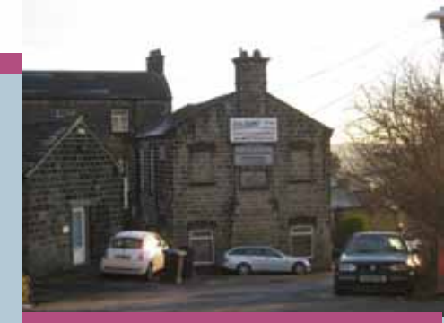
The former Friends School is one of many positive buildings in the conservation area.
