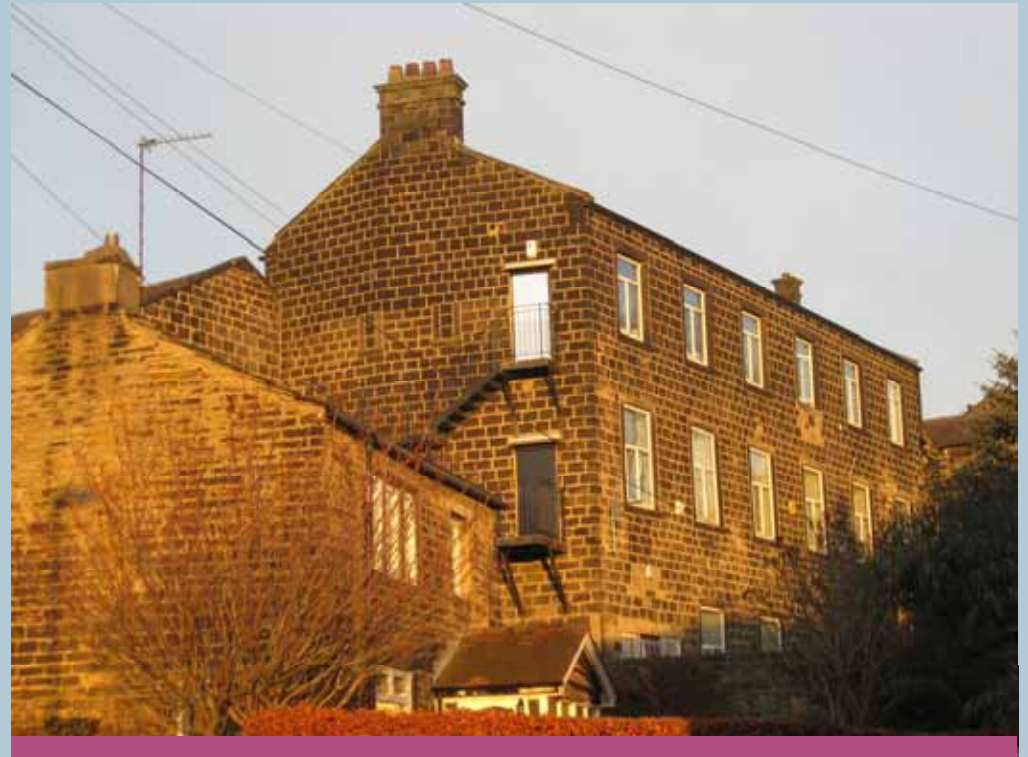
Any new build properties should take reference from existing positive architecture within the conservation area, particularly with regards scale, materials and detailing and respect important views.
