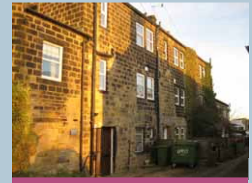
Three-storey weavers houses are common place in the conservation area, and may identify Low Green as a small centre for textile production in the early 19th century.
