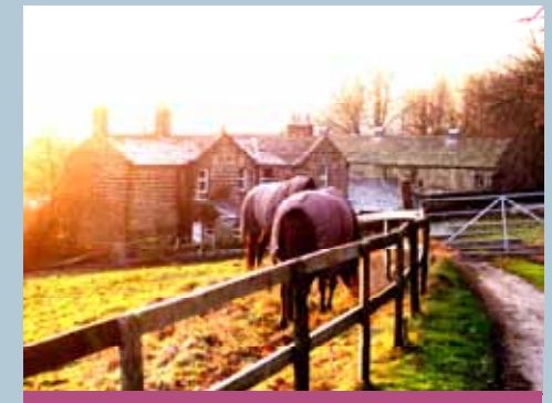
Rawdon Hall Farm is a very significant building in the conservation area, the majority of which dates from the late Victorian period
