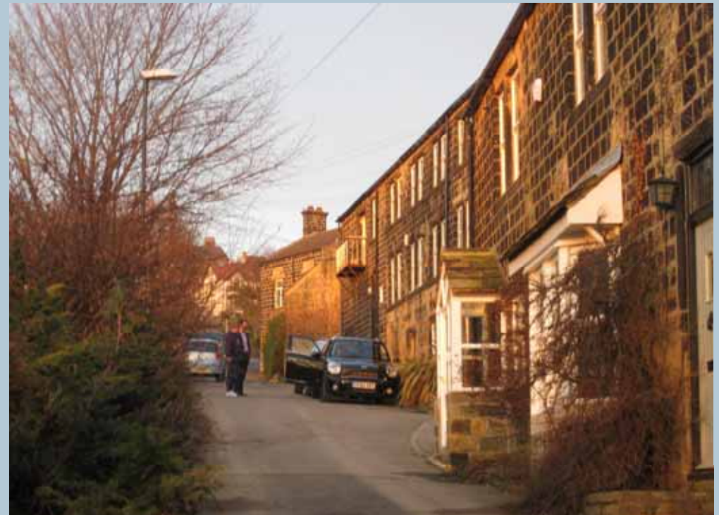
The back of pavement location of many of the historic buildings is an important characteristic in the conservation area. This creates a sense of enclosure, which contrasts with the surrounding open fields.
