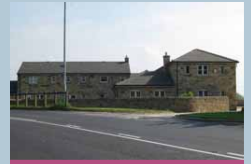
The redeveloped farmyard is the focus of initial views approaching the village from the north
