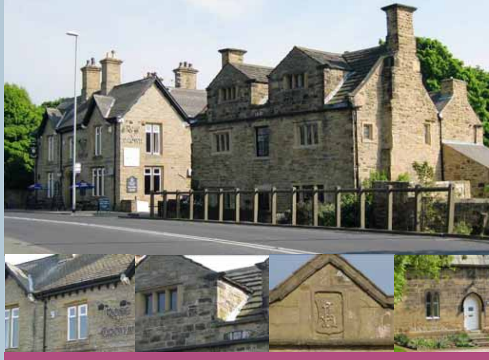
The old and new Rose and Crown - eaves details, reset 1642 rainwater head, 'JH' crest at Methley Villa and gothic details of the National school
