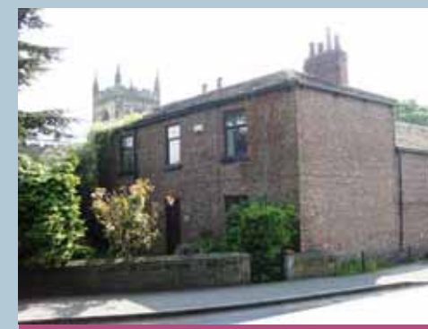
Brick is common, early 19th century handmade brick and stone slate roof, 30 Church Side
