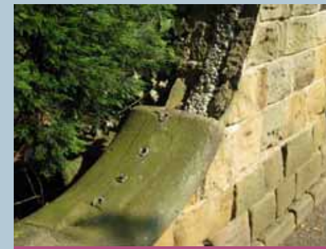
Reinstating lost historic details, such as boundary railings, would enhance the conservation area
