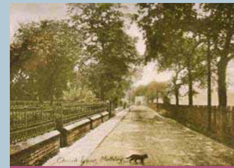
Historic photographs provide a good source of information for reinstatement schemes (Community Archives Group)
