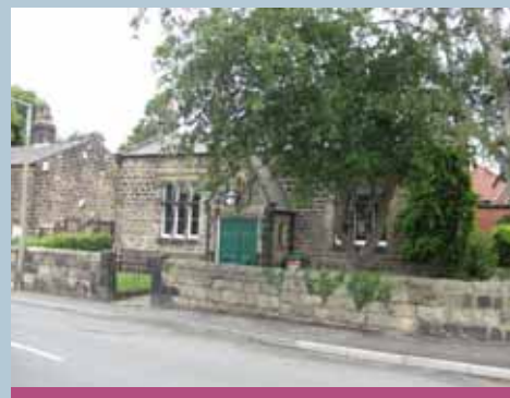
The Meanwood Institute, built c.1840 (Grade II listed)
