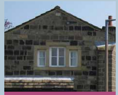
Simple but fine detailing on a property on Parkside Road
