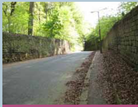
View 3—Looking north up Park-side Road
