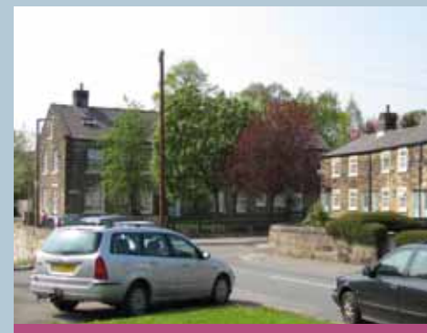
The Bywater buildings, Tannery Square (1852) (Grade II listed)
