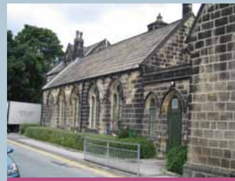
Gothic detailing on school building of 1840
