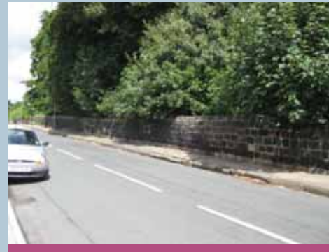
Boundary treatment, Parkside Road
