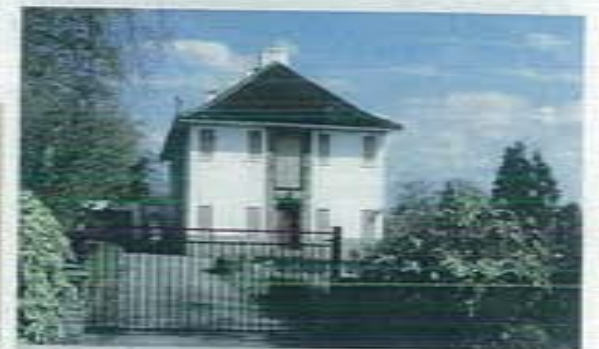
Boarded up Townend before demolition
