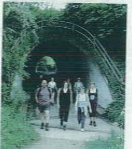
A6120 Ring Road, Adel Underpass
