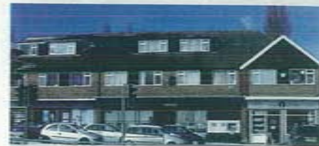
Otley Road Pedestrian Crossing by Nat-West Bank
