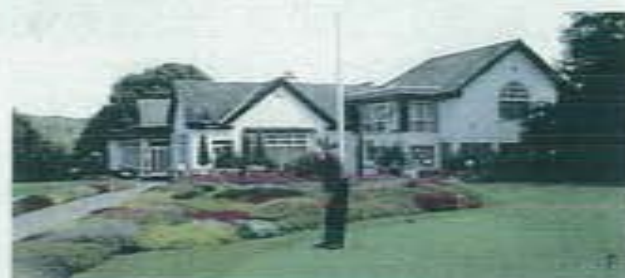
Club House, Back Church Lane, Adel
