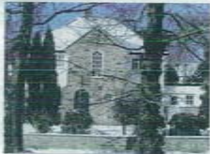
Adel Lane, west side
