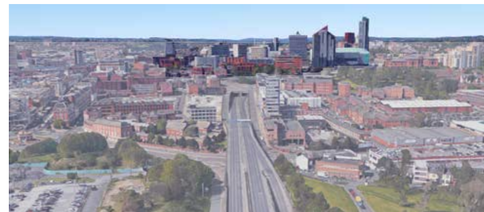
▼ Looking westwards above York Road (A64) - a group of tall buildings around the Arena
