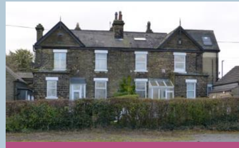
Coursed sandstone together with natural slate roofs, are the predominant materials of the conservation area.
