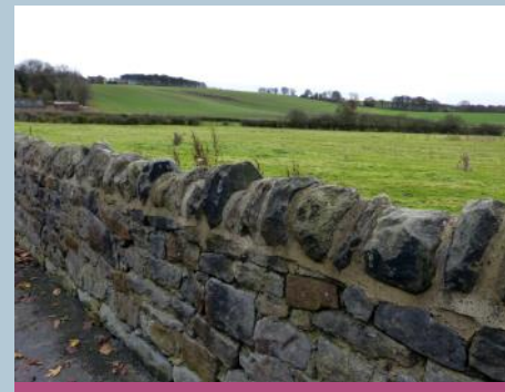
Sandstone boundary walls make a positive contribution to the character of the conservation area.
