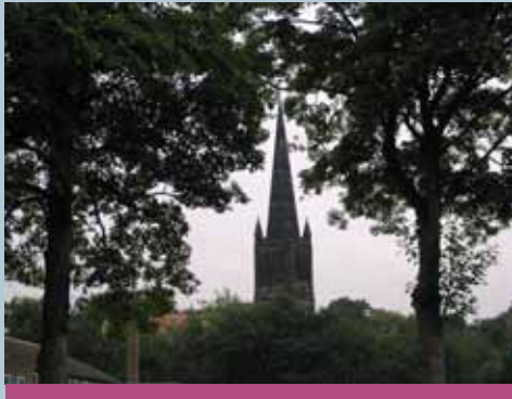
St Chad's spire is the principal landmark of the area
