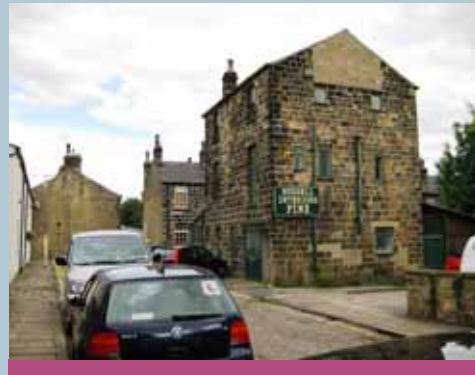
Industrial structure and York Stone paving, kerbs and stone sett road surface, Park Terrace
