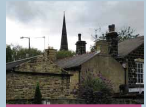
The roofscape is defined by simple pitched forms with prominent chimneys
