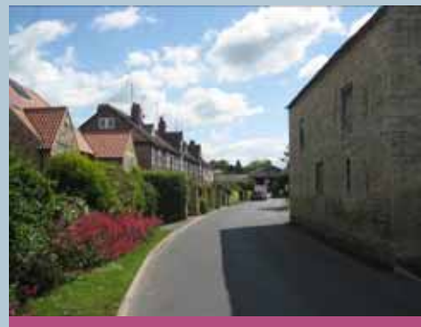
The lack of street clutter on back lanes enhances the character of the area.
