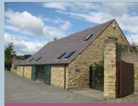
Recently converted "The Barn" is the oldest Secular building in Collingham, dating from the 1500s
