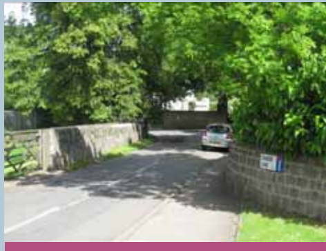
Stone boundary walls are important features which should be retained.
