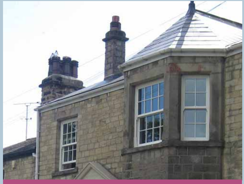
Historic windows, regularly coursed sandstone and chimneys are all traditional architectural elements which are positive to individual structures and the building stock as a whole.
