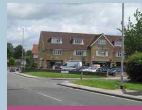
Exposed car parking in front of the shopping parade has a detrimental impact on the appearance of the conservation area.
