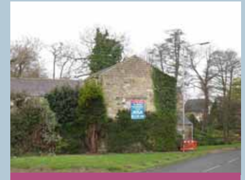
Collingham Mill is an important historic structure within the conservation area.
