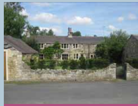
Buildings on the whole are two storey with regular fenestration. This consistent appearance is important to retaining the rural and historic nature of Collingham
