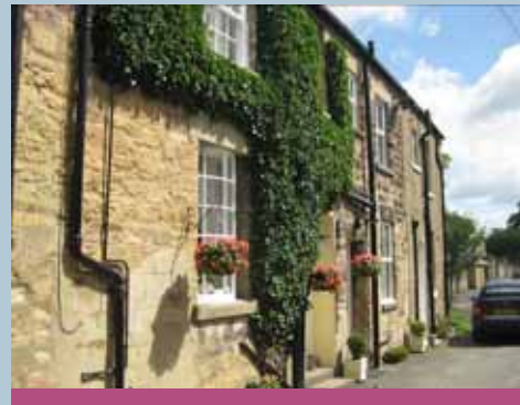
Coursed stone walling is the key characteristic of the buildings in Collingham
