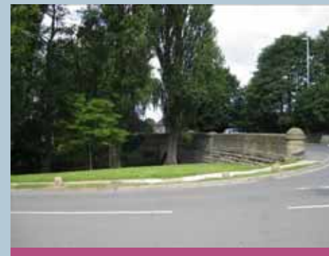
The bridge over Collingham Beck, built c.1790, is important for the development of Collingham.
