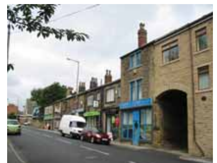
The majority of buildings in the Armley Moor/Far Fold character zone are built in stone
