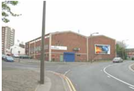
An industrial shed on the edge of the conservation area in need of improvement.
