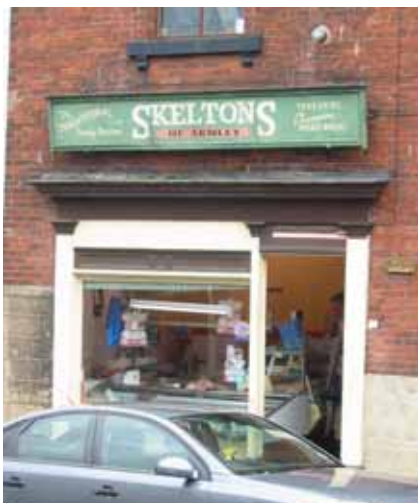
Original timber shop fronts survive on Town Street and Branch Road.
