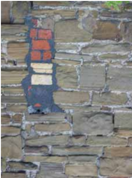
Local fine-grained sandstone was used as the main building material for walls and the roofs in Armley until the middle of the 19th century.
