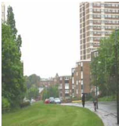
The 1960s public housing at Far Fold destroyed Armley's intimate scale and spatial structure.
