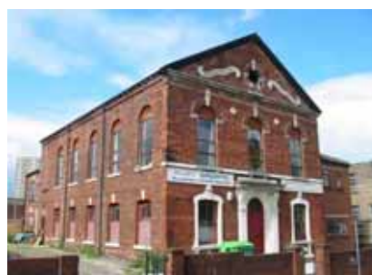
The former Temperance Hall and Mechanics' Institute.
