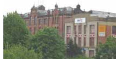
Former Scotch Foundry.
