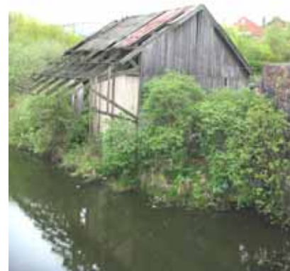
Loading bay below Scotch Foundry.
