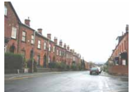
Superior terraced housing on Wesley Road.
