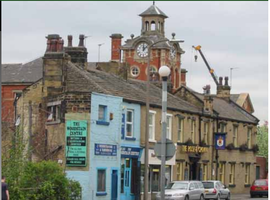
Armley Road looking east showing common materials and building styles.
