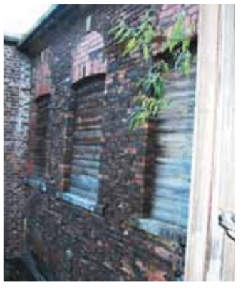
Details of the original building are still visible
