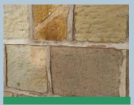
This cement pointing is actually causing damage to this soft
