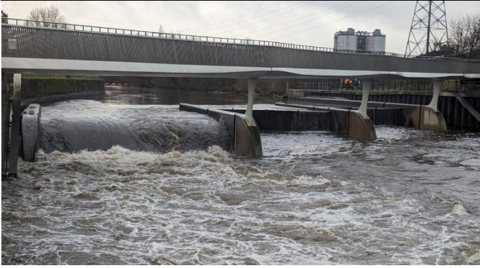
Figure CC2: Knostrop – weir down (FAS1)
