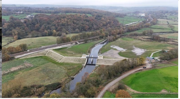
Figure CC3: FAS2 Flood Storage Area, Calverley
