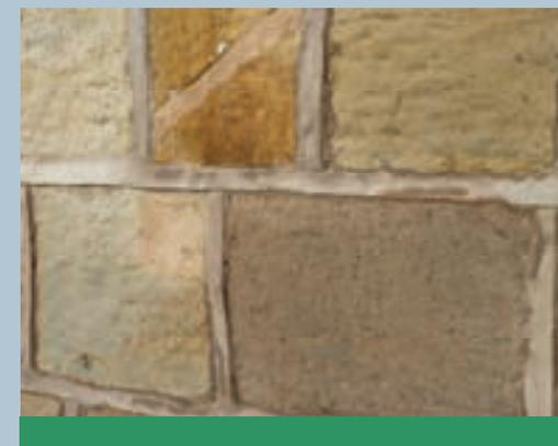
This cement pointing is actually causing damage to this soft sandstone.
