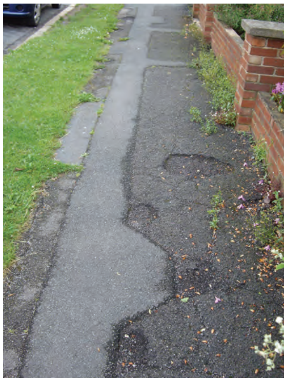
Fig. 5.7 Irregular footpath due to degradation
