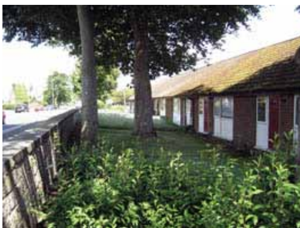
Poor relationship: Beech trees at 4m from the front of a dwelling are overbearing and cut out light
