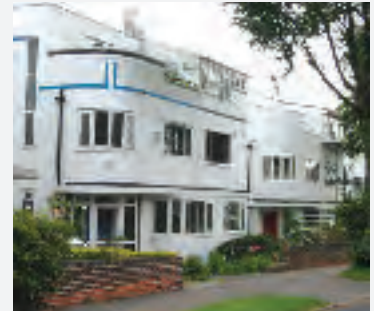
MODERN MOVEMENT STYLE OF 1930S Provides light, attractive living space
