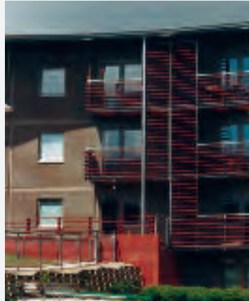
RECENT LOW RISE BLOCK OF AFFORDABLE FLATS TO RENT Attractive, award-winning design
