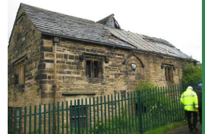
Stank Hall Barn, Beeston
