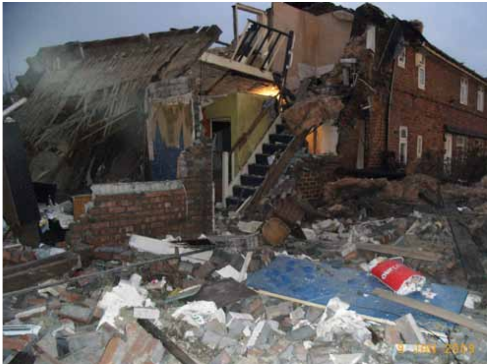
Figure 1. This is the site of a gas explosion in a terraced property in Middleton. The explosion occurred at around 4 pm on a Friday afternoon and miraculously there were no serious injuries despite the house being located on a busy main road. The explosion was caused by leaking gas and was triggered by the occupant of the house lighting the cooker. The occupant was treated in hospital for minor injuries but made a full recovery. The house at the centre of the explosion, along with the property next door, required demolition.
