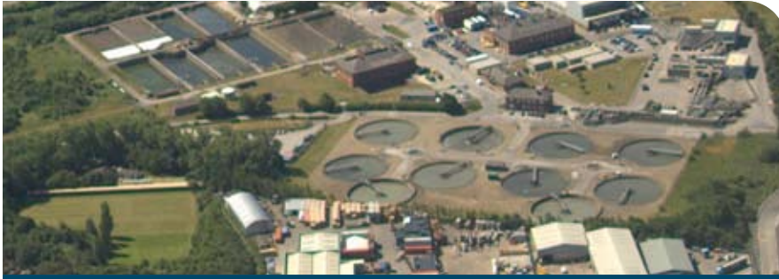
Lower Level Works at Knostrop
