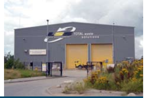
Recycling Centre, Cross Green
