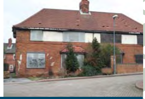
Boarded up houses, Halton Moor Road
