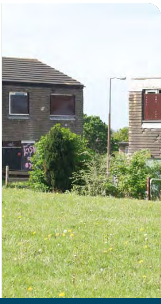
Housing to be cleared, South Parkway - Seacroft
