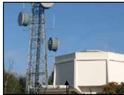
22.5m high base station which has a lattice structure.
