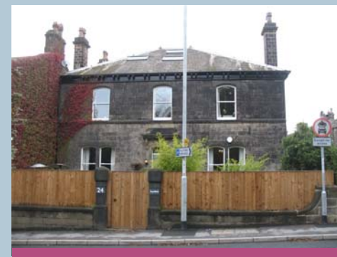
Inappropriate boundary fence. Railings would have been preferable.
