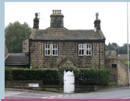
The Springwood group of cottages forms part of an important gateway.
