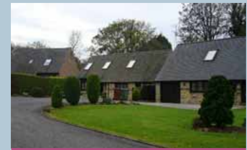
Oulton continues to evolve. There has been a substantial amount of 20th and 21st century residential infill development, such as here at Woodland Park
