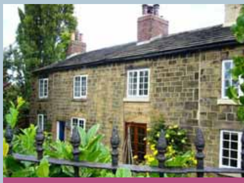
Some historic railings survive, such as here at Leeds Road
