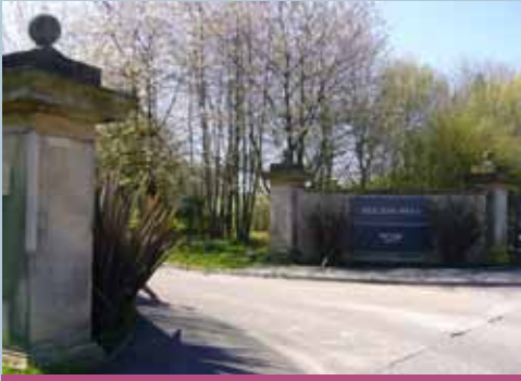
Gateways and boundary walls are distinctive features of Oulton Park
