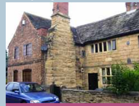
9-13 Farrer Lane, 16th century or earlier farmhouse with timber-frame cased in sandstone and handmade brick
