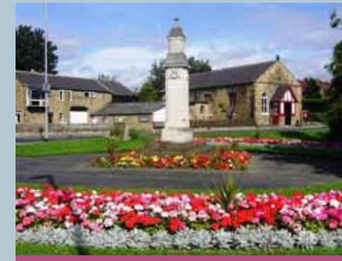
Important gateway to the village proposed for inclusion in the revised conservation area (Area C)
