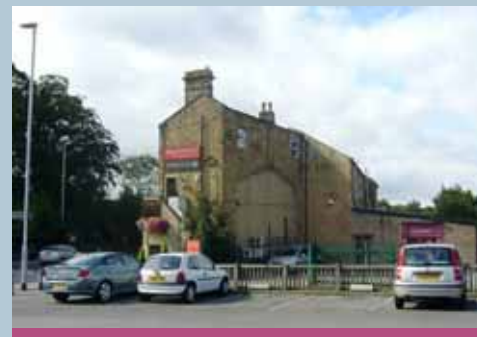
Improved boundary treatments to the Old Mason's forecourt could enhance the conservation area
