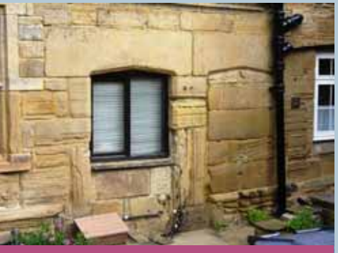
Tudor-arched lintels are a typical detail of the 16th and 17th century buildings, including this example at 9-13 Farrer Lane
