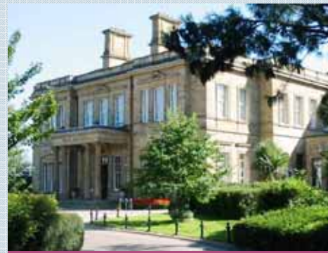
Oulton Hall, north front entrance by Perkin and Backhouse 1851-4
