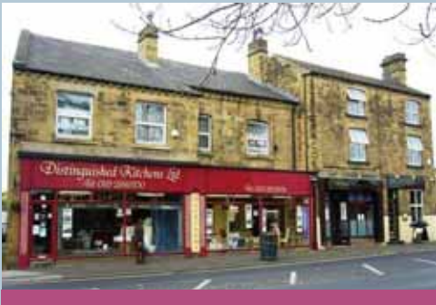
The village has a number of shops including this group set within late 19th century buildings, Aberford Road
