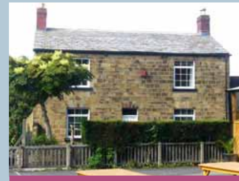
Plainly detailed 18th century stone house with sandstone voussoirs to window and door lintels, 9 Manor Lane
