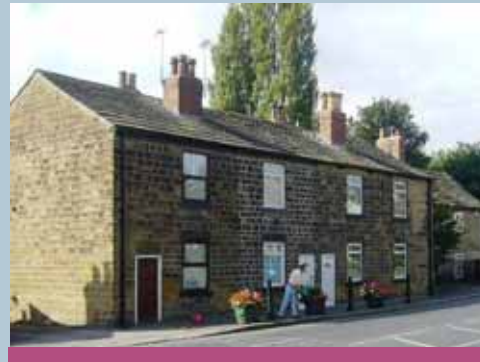
Street fronting cottage rows are an important architectural group such as 8-12 Calverley Road
