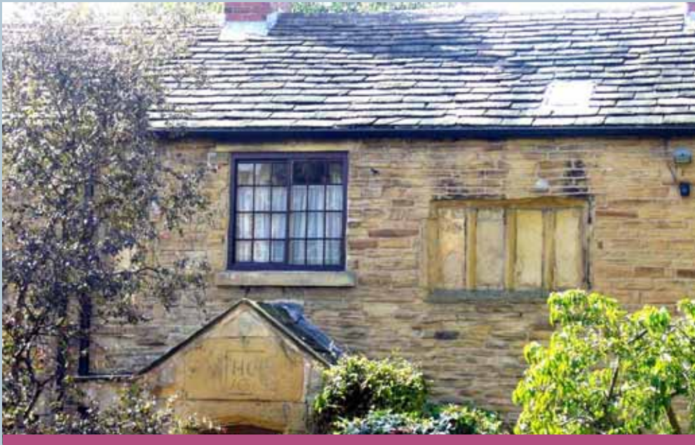
The patina of age, richness of texture, quality of materials and surviving historic detail such as at the 17th century Ivy Cottage, Calverley Road are essential elements of the conservation area. Date stone reads 'HC 1699'
