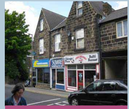
Inappropriate shop fronts on Town Street
