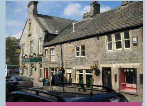
Example of a once long vacant property on Town Street (far right). Now being refurbished and brought back into reuse.
