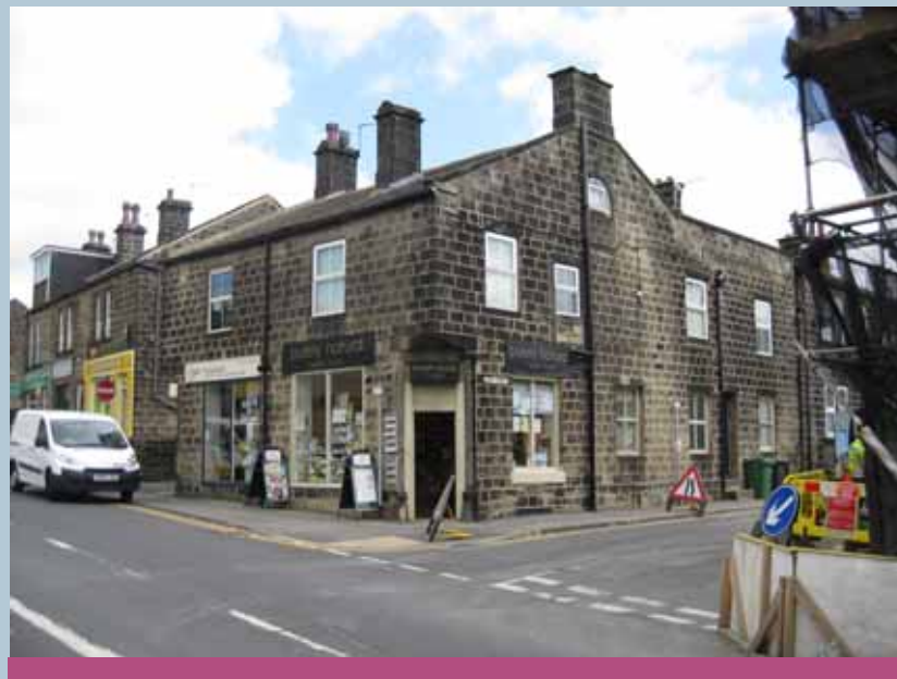
Interesting details such as corner doorways should be retained
