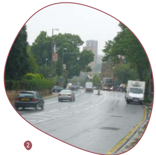
2 View downhill along Chapeltown Road
