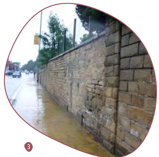
3 Stone front garden walls
