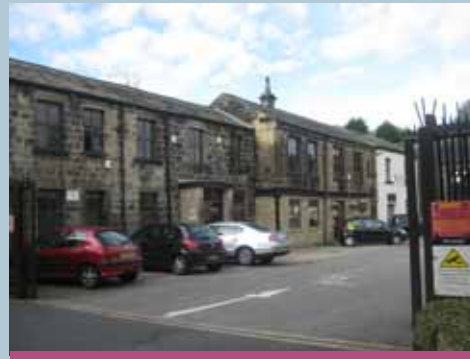
The Bagley area contains some buildings extremely important to the character and history of Farsley, including Springfield Mills.
