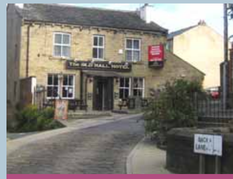
Sympathetic street surfacing on Back Lane improves the character and appearance of Farsley, and should be employed where possible elsewhere in the conservation area
