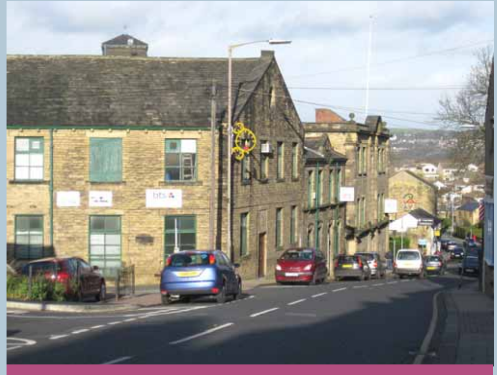
The remaining industrial architecture is very important to the character, appearance and history of Farsley. With so much demolished, retaining what is left would be of positive benefit to the village
