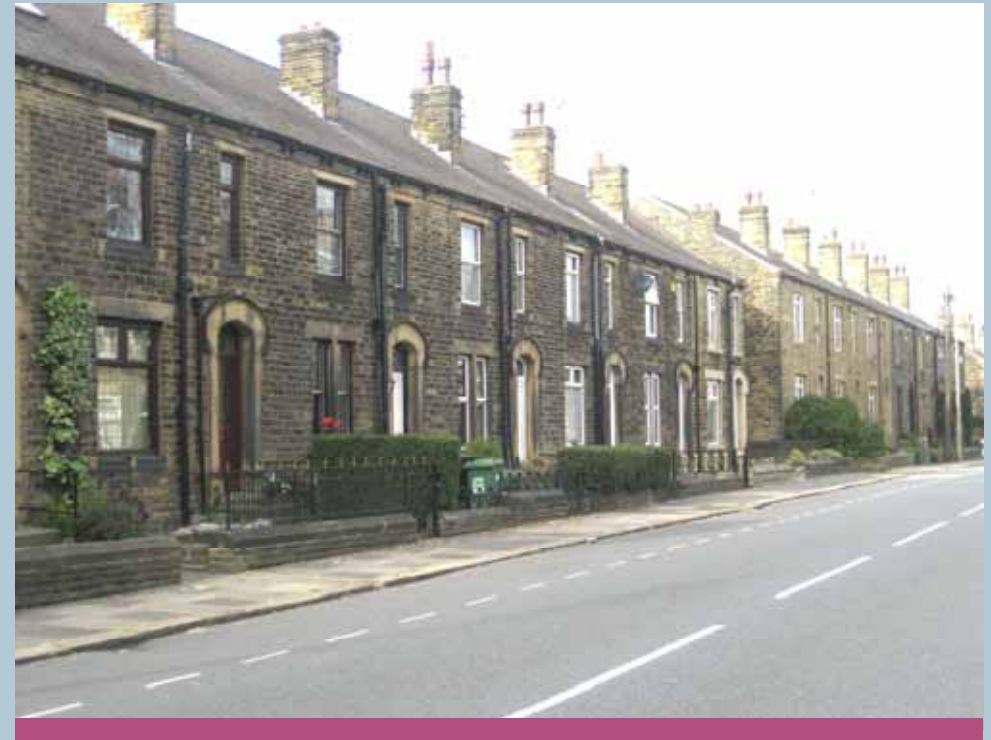
Terrace rows dominate large parts of the conservation area. Traditional coursed sandstone, Welsh slate and chimney stacks and pots are important characteristics of a terrace row.
