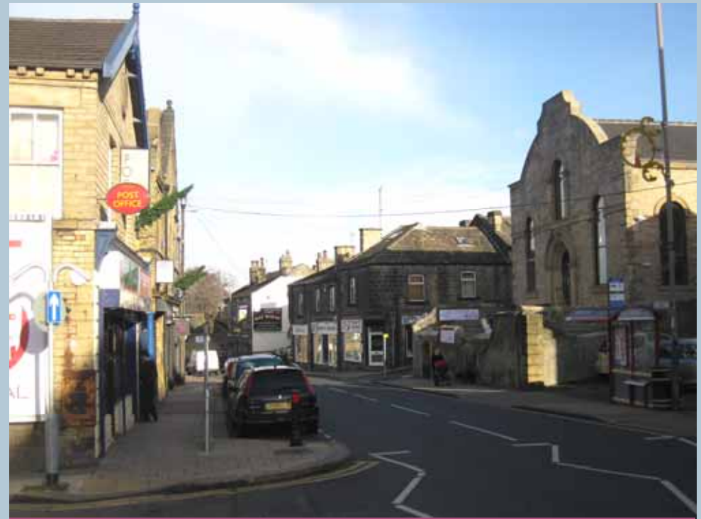
Variation of architecture helps define the character. This is a positive attribute which emphasises the piecemeal development of central Farsley.
