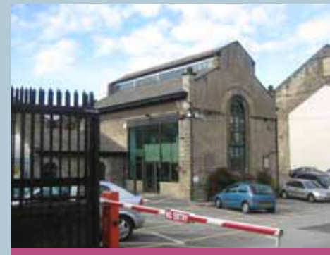
Springfield Mills has retained many parts of the historic mill, which increases its importance.
