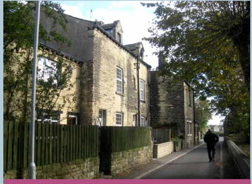
Dominant buildings and stone boundary walls enclose the streetscape around much of Farsley.
