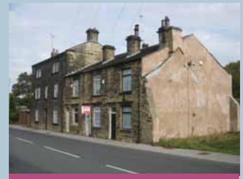
18th historic buildings further emphasise the importance of Bagley as a settlement predating Springfield Mill.
