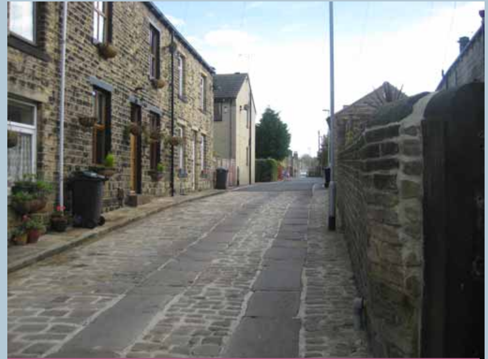
Resurfacing works on Prospect Street (above), High Street and Back Lane have had a positive impact on the character and appearance of the conservation area. This approach sets a standard for the public realm of the area.
