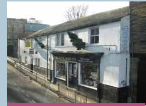
Traditional shopfronts enhance the character of the conservation area.
