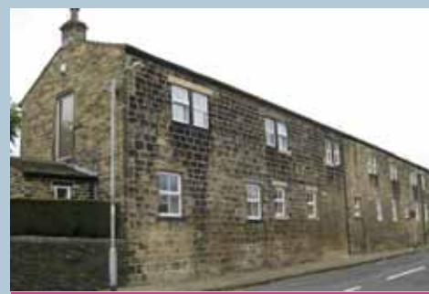
Rushton Street. Former woollen waste store, with taking-in door to first-floor visible in gable end.
