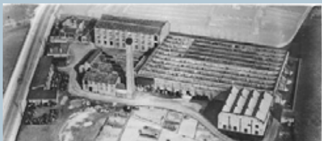
Lydgate Mills, aerial view. The mill was demolished in the 1970s and housing built in its place.
