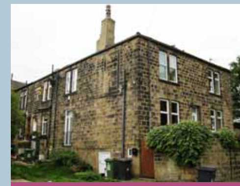
15-16 Chapel Street. The blocked first floor doorway indicates that this building provided living accommodation downstairs and working space upstairs.
