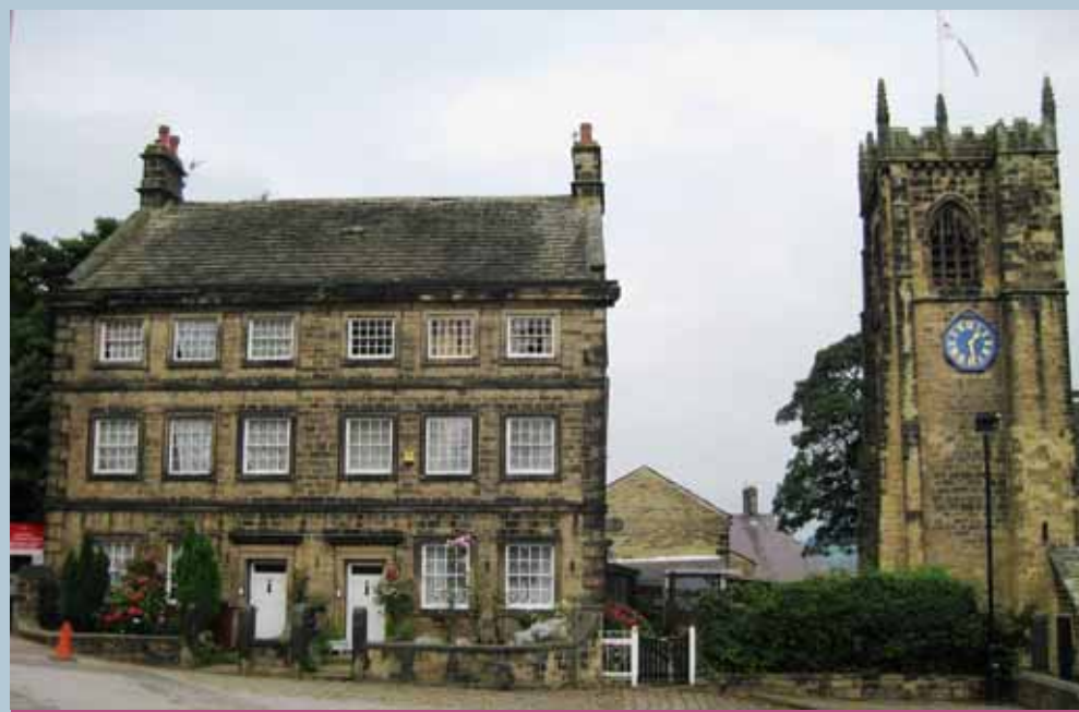
1 & 3 Church House, Town Gate. An unusual example of semi-detached 18th century houses, listed grade II*, next to the Grade I listed church.
