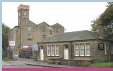
Ravenscliffe Mill, another large late-19th-century woollen mill, which has been converted to light industrial use. The survival of the mill buildings makes a considerable contribution to the character of the area.
