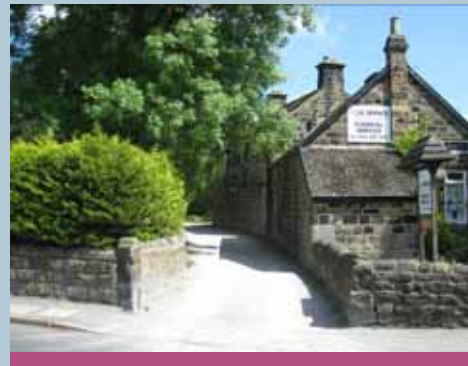
Lower status structures also employ regularly coursed stone in both buildings and boundary walls
