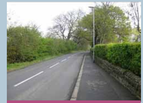
Generally signage, street furniture and surface treatment is ordinary, such as here at Church Lane.
