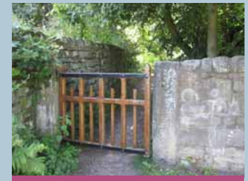
Footpaths, such as the lane that runs off Back Church Lane and towards the church are important features in the conservation area
