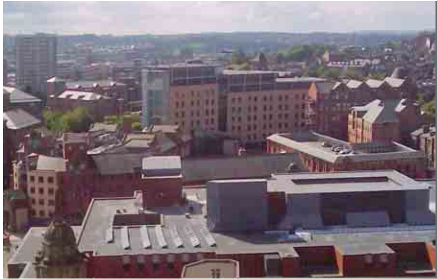
Solar panels on the roof of Leeds County Courts
