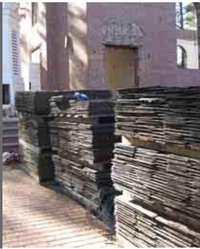
Re-using old roofing slates
