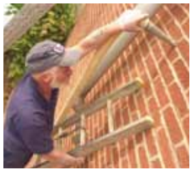
insulating the walls
